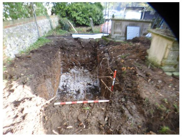
Plate 9. Excavation for new septic tank
